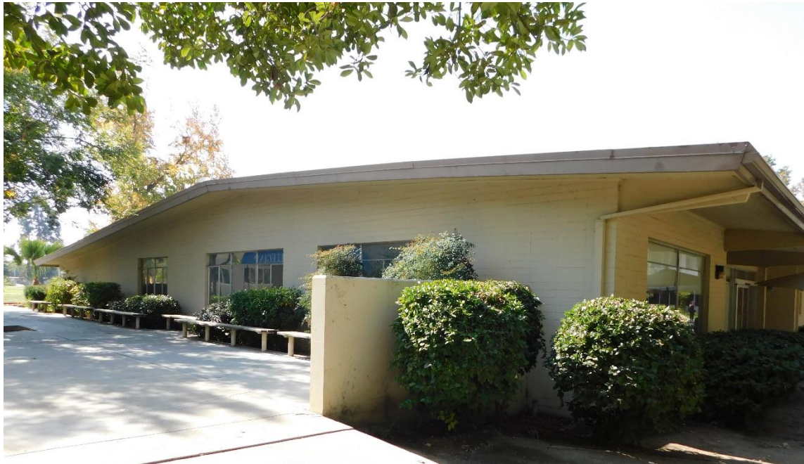
East Elevation, view to southwest, DSCN2201
