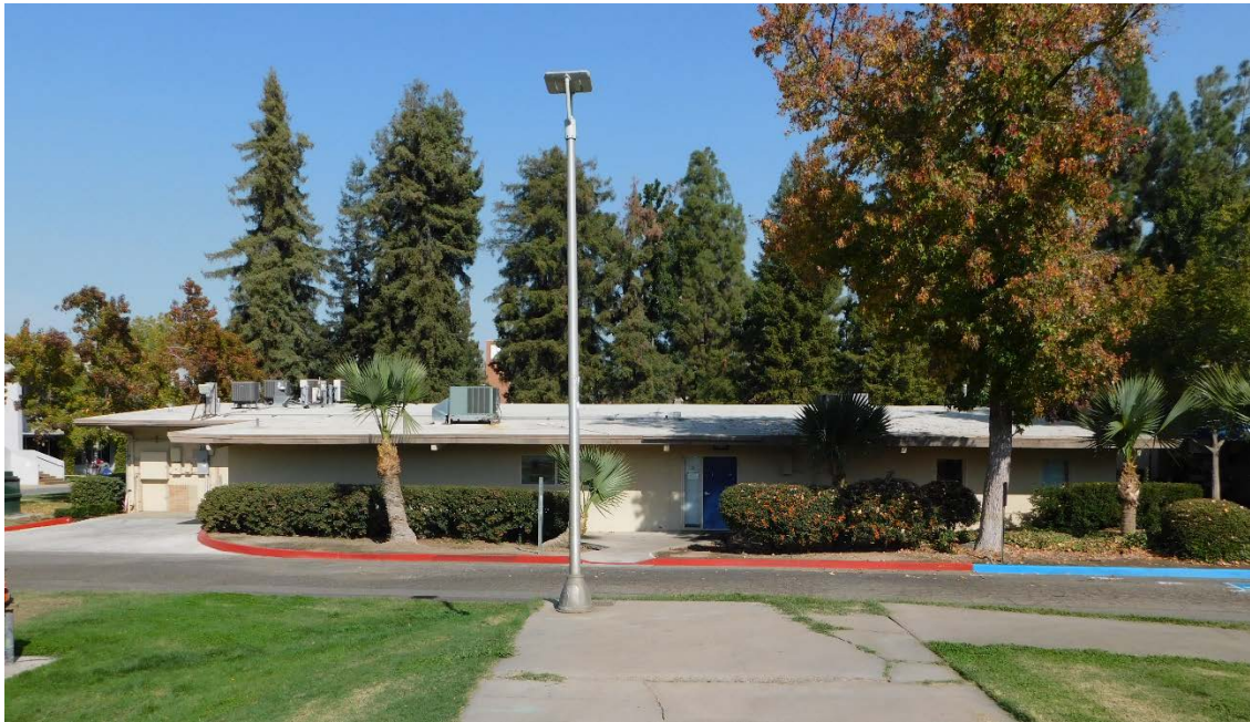
Figure 5. South (Rear) Elevation, view to north, DSCN2171
