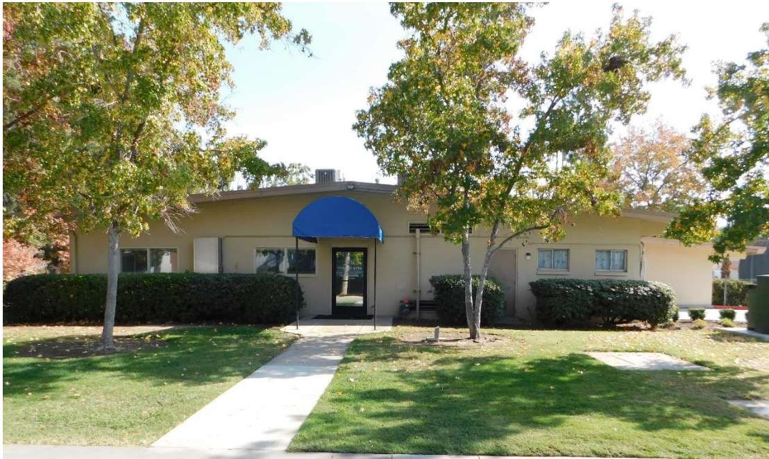
West Elevation, view to east, DSCN2277
