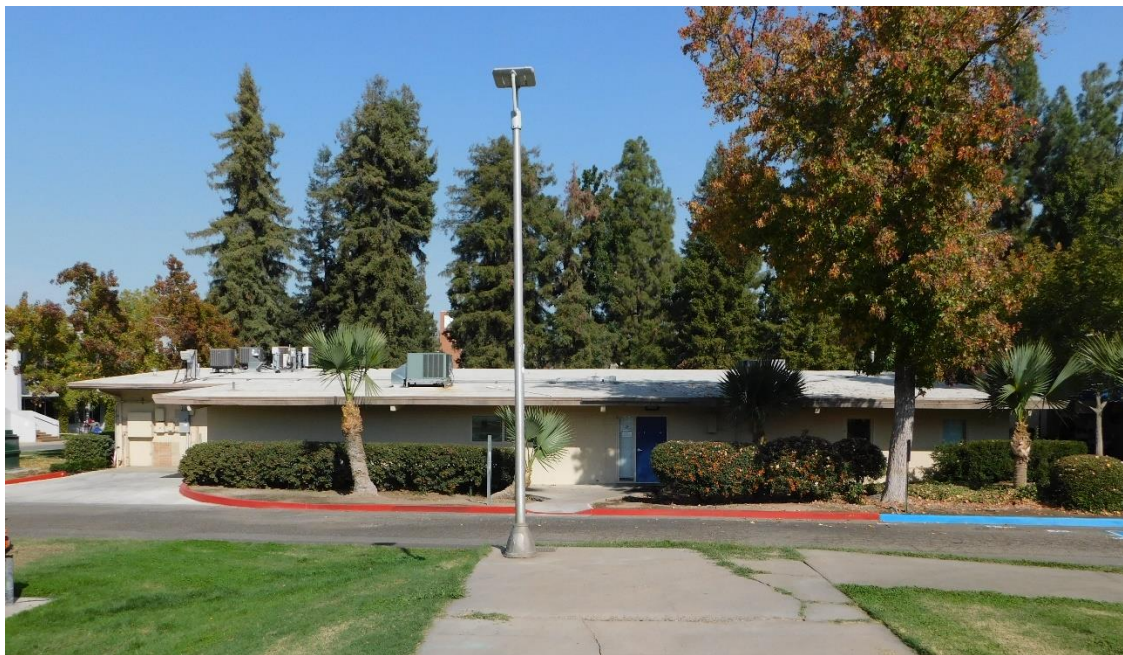
South (Rear) Elevation, view to north, DSCN2171
