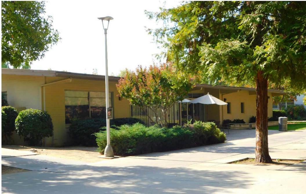
Figure 3. North (Main) Elevation, view to southwest, DSCN2275
