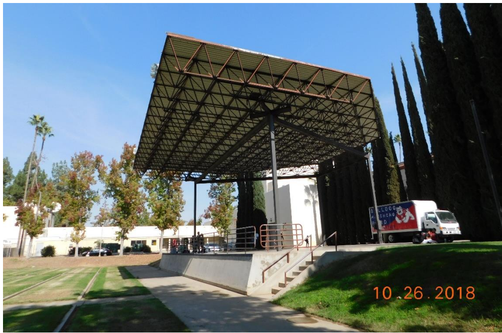
Side View of Truss System, view to northeast, DSCN2206
